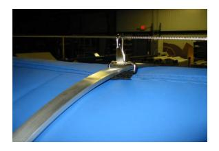
After both ends are connected even out hanger so it is centered And clip snaphook to cable
